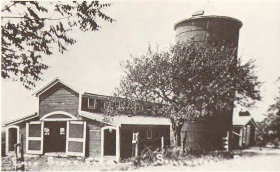
From the top of this silo, Mr. Emin could survey the Smithfield countryside. The barn, part of the Emin farm, is no longer standing.
