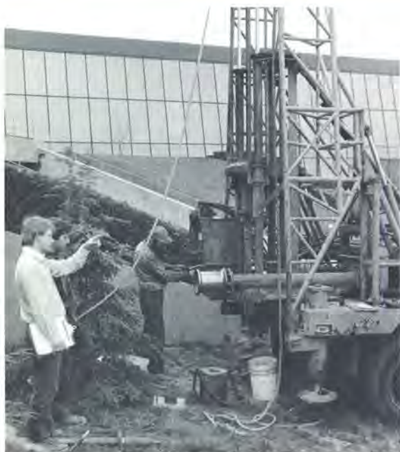
Drilling to gauge spread of oil spill.
