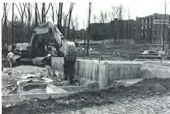
Backfilling a foundation for the Townhouse.
